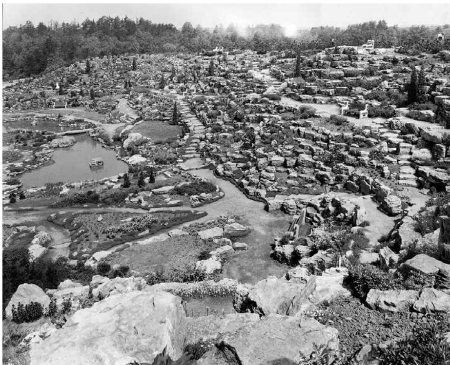
Rock Garden under construction, 1931
