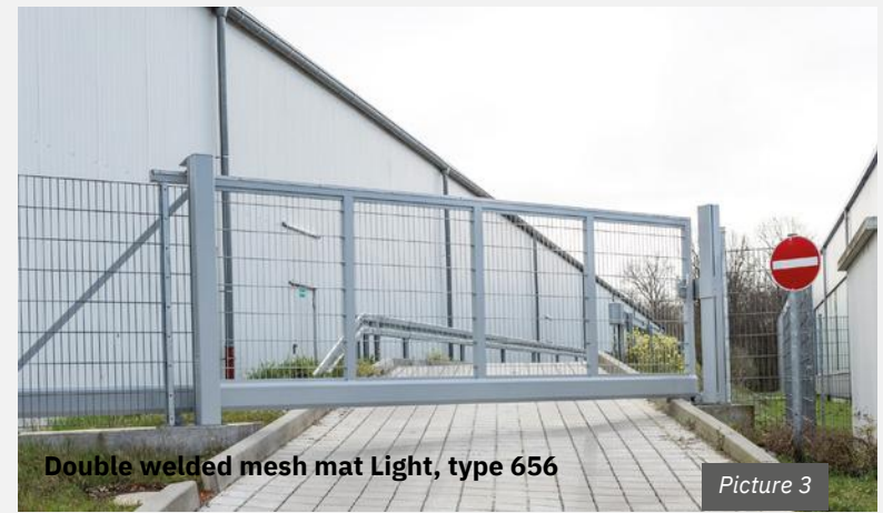
Bar 30 x 30 mm with diagonal bracers
