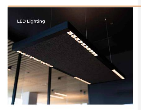
Low-power LEDs are used for all office lighting. Special sensors activate lights based on the presence of people and adjust intensity according to natural light.
