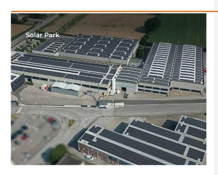
A new photovoltaic system was installed at the end of 2023, complementing the existing one from 2012. Covering 20.000 sqm (215,000 sqf) of roofs, with 5.000 modules and a peak power of around 2 megawatts, it has become fully operational during 2024 and is meant to serve about 80% of the company's electrical needs.
