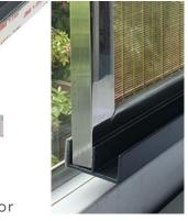
With no mullions or brickwork to install the shading onto, 3M VHB Tape was used to fix to the glazing.
