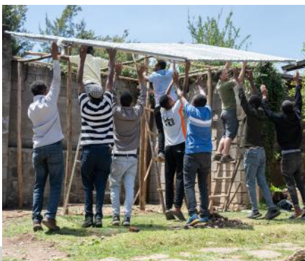
GULELE CENTER Plastic Roof Covering
