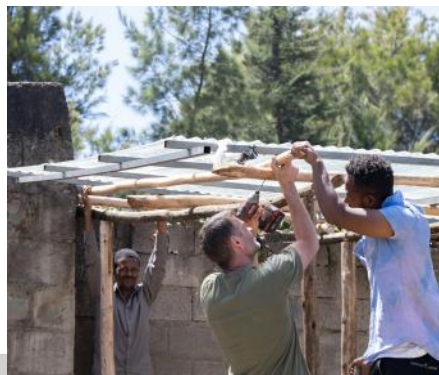
GULELE CENTER Working together
