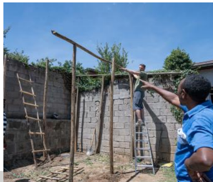
GULELE CENTER Outdoor shelter construction
