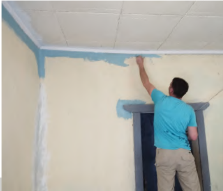
KALITY CENTER Painting & Plaster Repairs
