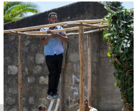
GULELE CENTER Building the frame!
