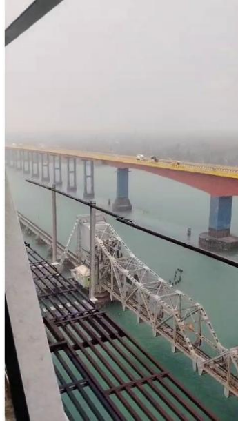
Unexpected Rain interruptions
