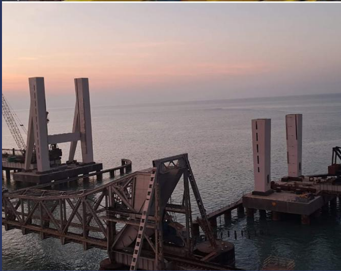
Different stages of the lift shaft construction
