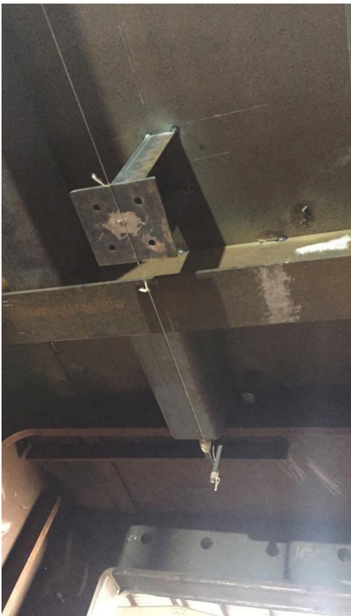
Plumbing guide bracket positioning during shaft fabrication
