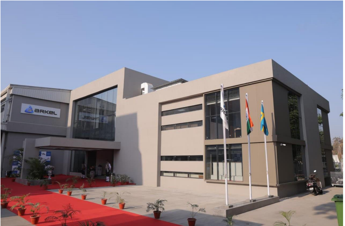
Spanning 1,35,000 ft 2 , the Arkel Electronic India Pvt. Ltd. facility in Vadodara, Gujarat, is built to deliver scale with precision.
