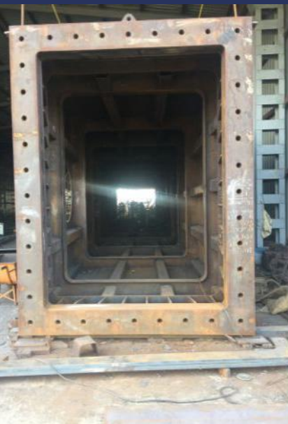
Fabrication of the shaft structure at the yard
