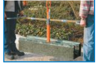
• Posa cordoli e canali Kerb and curbstone laying
