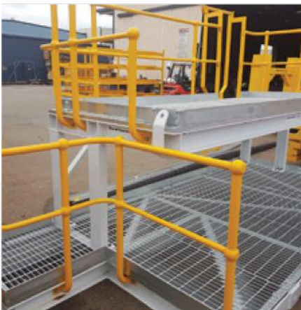
Handrail and Floor Grating
