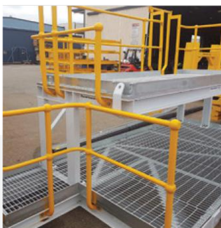
Handrail and Floor Grating
