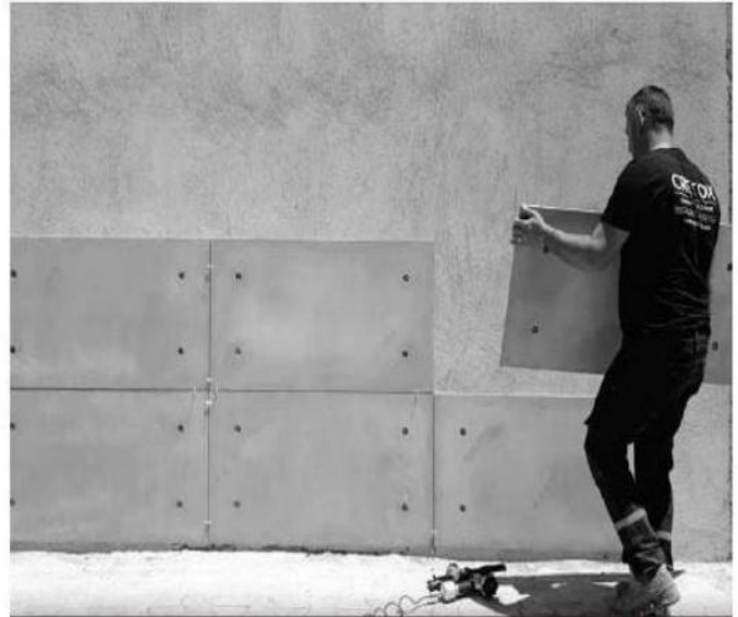
GLUE TO RAW WALL + MECHANIC SUPPORT / EXTERIOR 1
