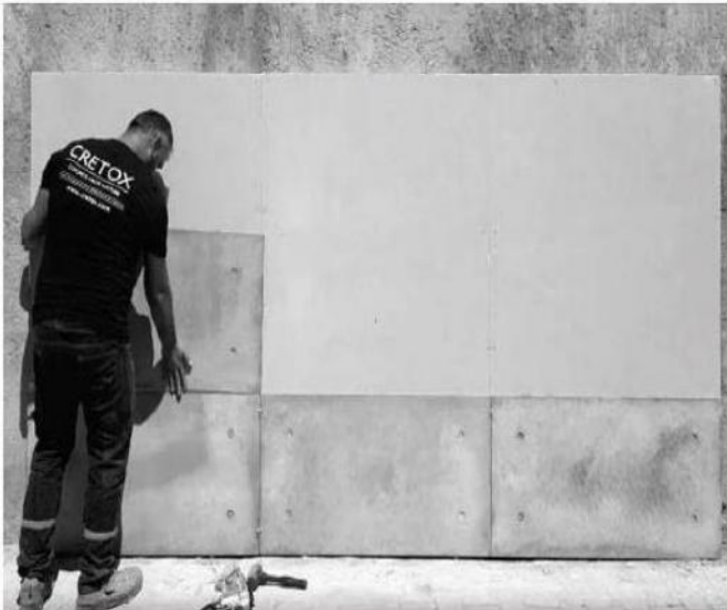
GLUE TO EXTERIOR BOARD + MECHANIC SUPPORT / EXTERIOR 2
