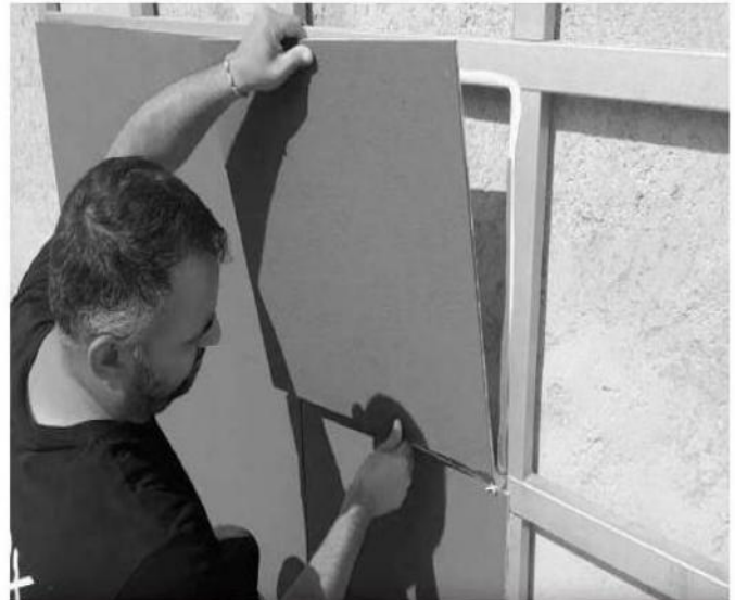
GLUE TO METAL FRAME + MECHANIC SUPPORT / EXTERIOR 3
