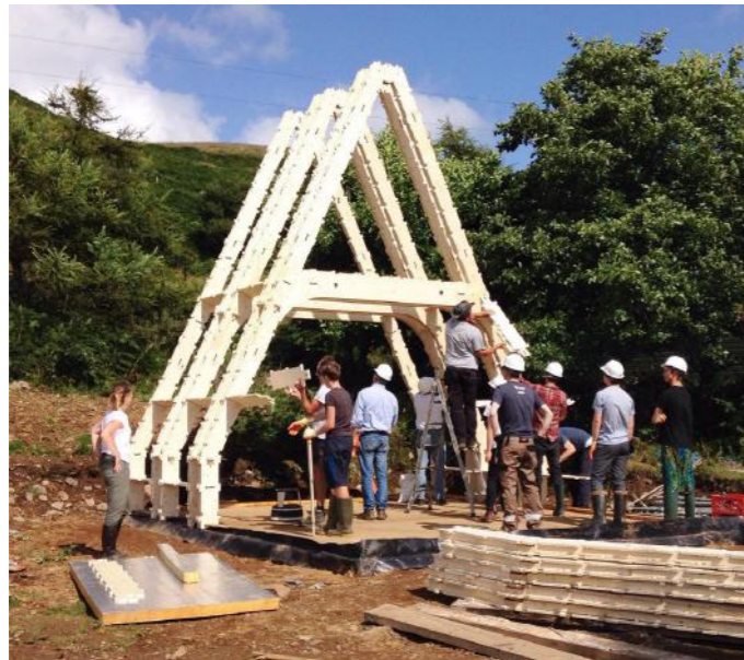
📷 A-Barn in construction. Image courtesy of WikiHouseFoundation.
