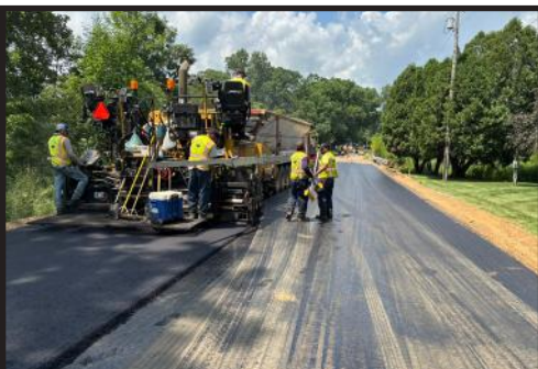
HMA paving on U Avenue
