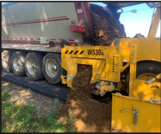
Placing shoulder gravel on XY Avenue
