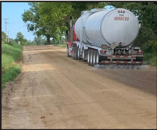
Applying dust control on 40th Street
