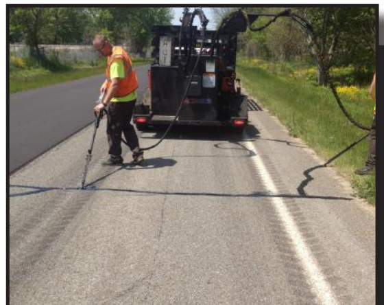
Crack fill on K Avenue
