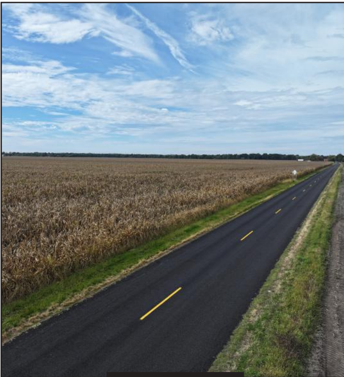
Chip seal on YZ Avenue
