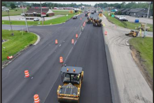
HMA paving on Sprinkle Road
