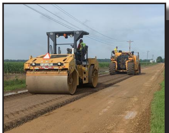
Pulverizing XY Avenue
