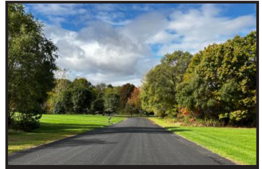
Chip seal/fog seal on Stoney Woods Drive
