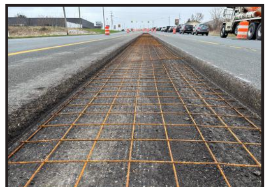
Concrete work on Sprinkle Road
