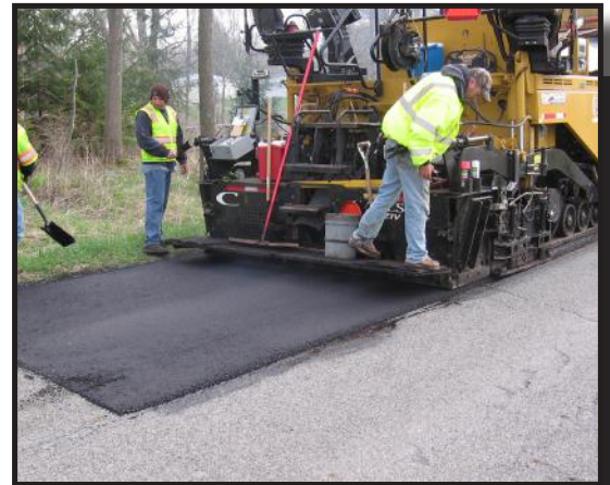
HMA wedge on V Avenue
