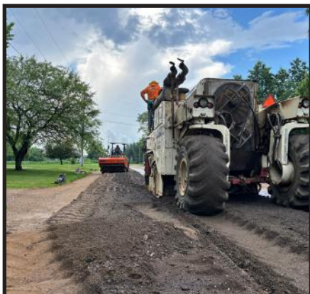
Construction on U Avenue
