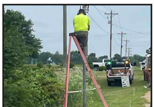
Traffic signal maintenance
