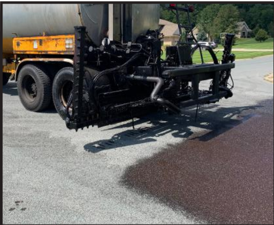
Fog seal in Oshtemo Township
