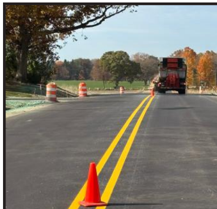
Pavement marking on Q Avenue
