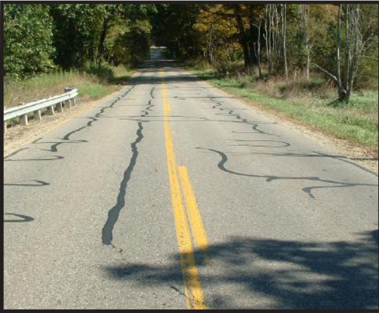
Crack seal on O Avenue
