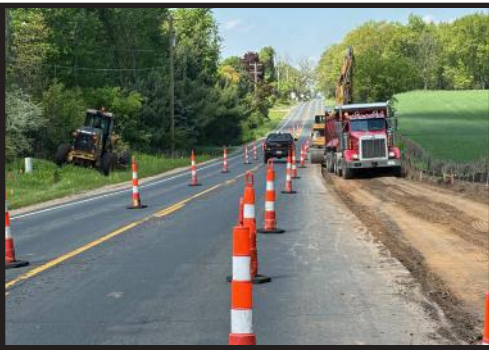
Widening on G Avenue
