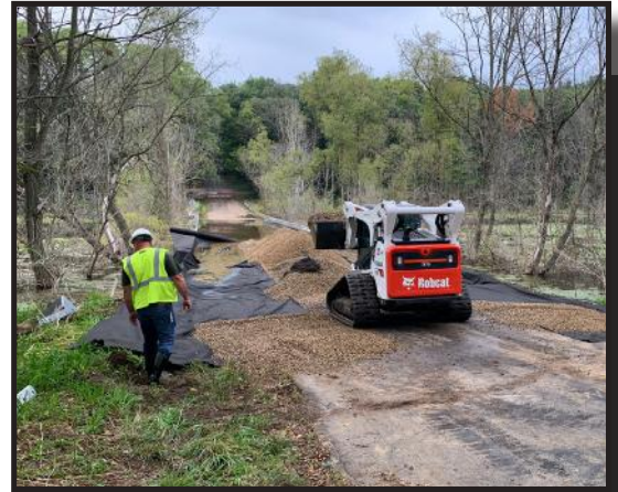
Aggregate lift on 8th Street bridge
