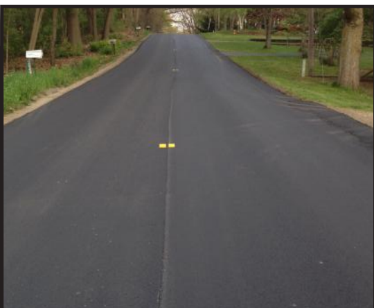
HMA paving on JK Avenue
