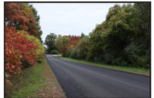
Chip seal/fog seal on DNR Street
