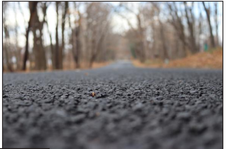
Chip seal/fog seal on B Avenue
