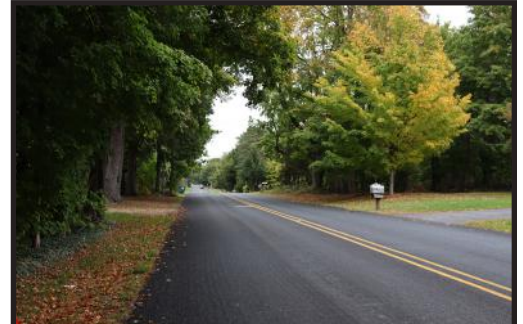
Chip seal/fog seal on Chadeau Avenue
