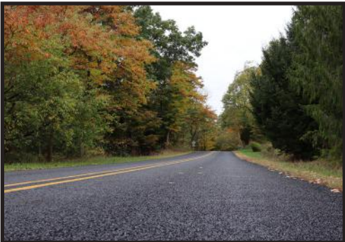
Chip seal/fog seal on RS Avenue
