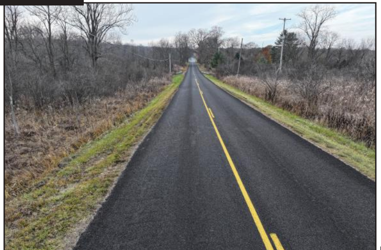
Chip seal/fog seal on B Avenue
