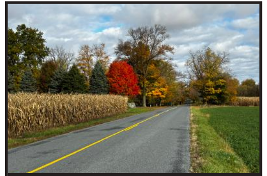
Chip seal on 38th Street
