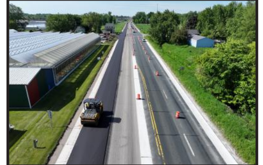
HMA paving on Sprinkle Road
