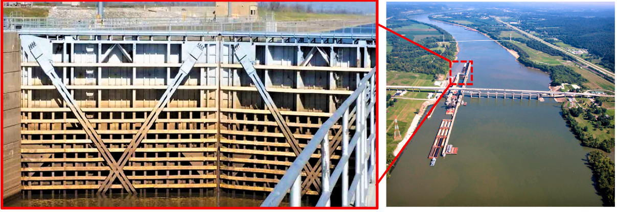
Fig. 1. An example of a lock and miter gate system.
