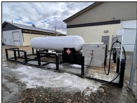
Propane Filling Station with Tank On Skid
