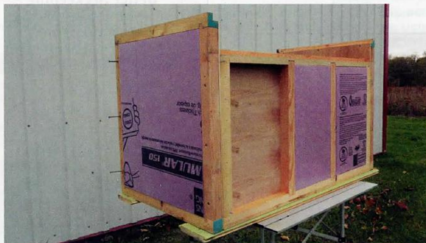
Internal construction of insulated horizontal hive." (Author's photo)
