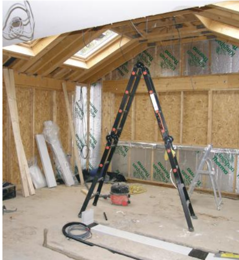
Construction of new garden room with Velux windows.
