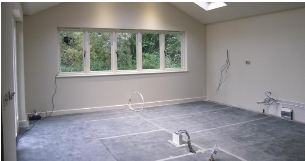
First fix completed with services positioned correctly ahead of kitchen installation.
