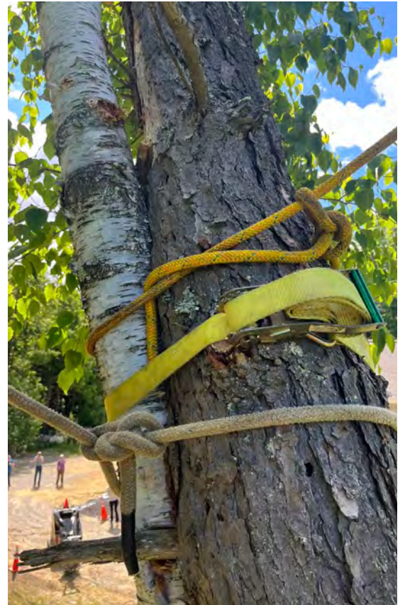
Photo 9: Rigging set at the location where the hemlock and birch were in contact with each other. Note how the load binder strap and rigging lines were secured around both stems.
