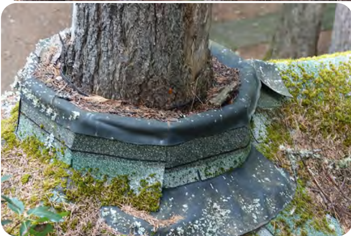
Access by suspension bridges supported by steel cables. BELOW: Rubber gaskets divert most rainwater to the exterior of the roof.
