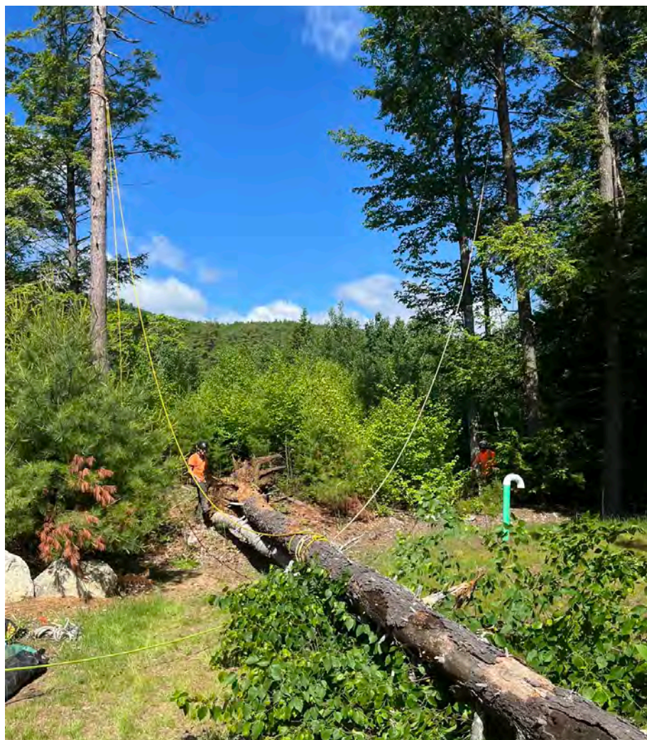
Photo 12 : Both trees were lowered to the ground safely, adjacent to the leach field and with zero impact.
