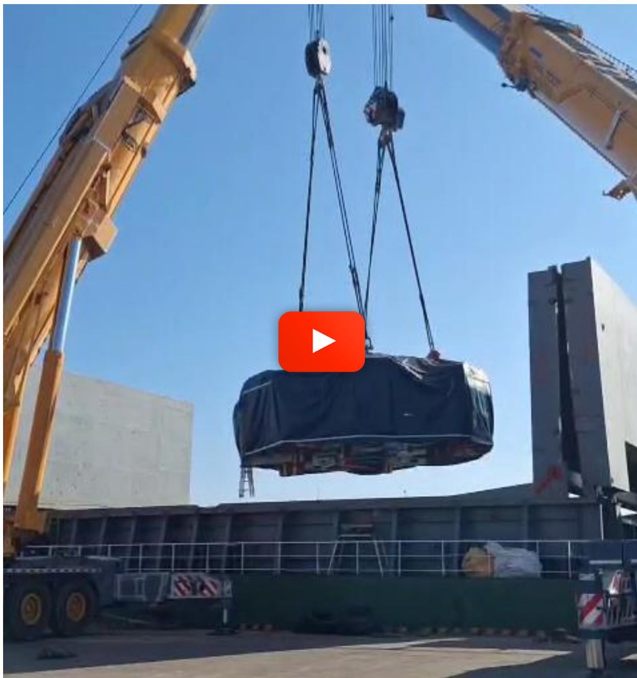
The cargo included one piece that weighed 147 metric tons and six pieces that weight 47 metric tons each.
