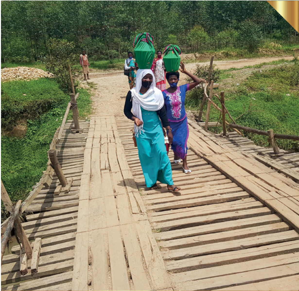
This is a picture from Rwanda. People used this rickety timber bridge to cross a river to get to the market. It washed away frequently during floods.
