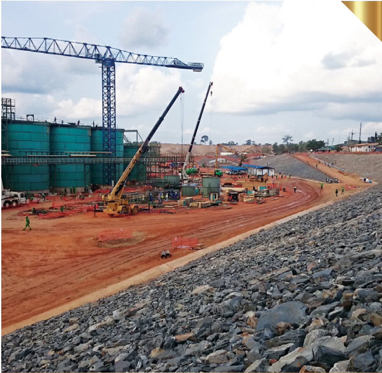
iCU at Asanko Gold Mine
