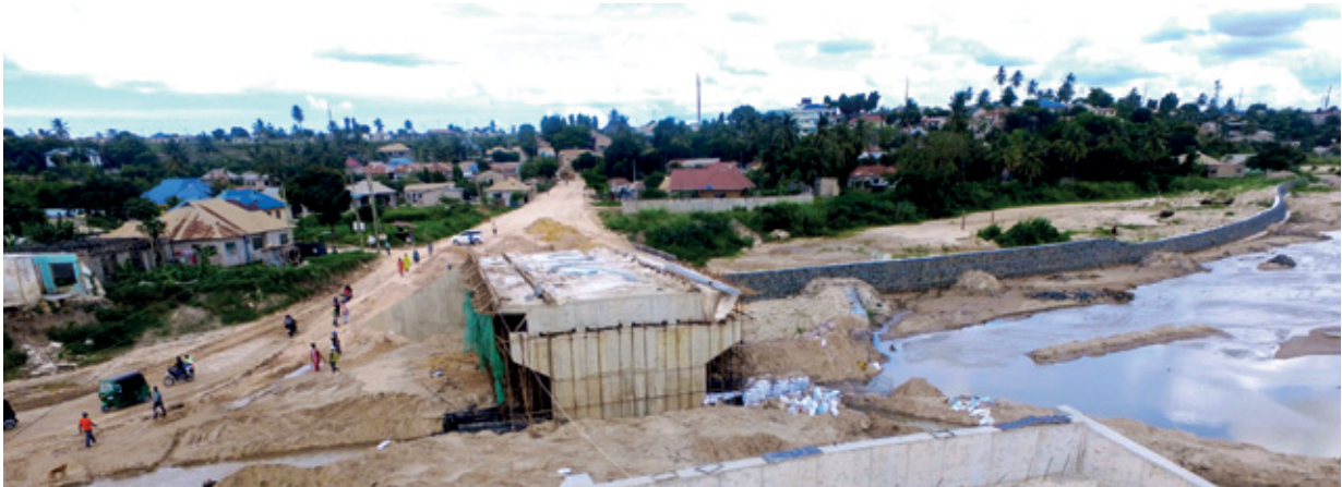
Dar es Salaam - Zimbili bridge construction
