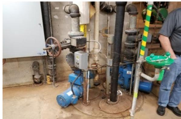
Figure 3 . Sanitary waste ejector pump
