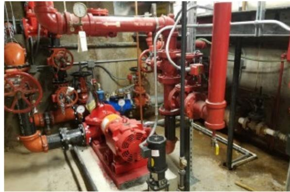
Figure 1 . 30 HP, 208 V, 3 PH, Fire Pump installed in 2016
