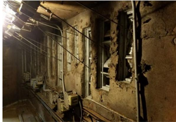
Figure 8 . Interior of original basement AHU insulation spalling
