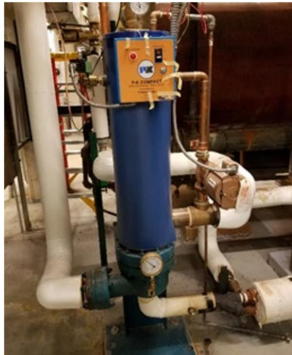
Figure 2 . Semi-instantaneous water heater
