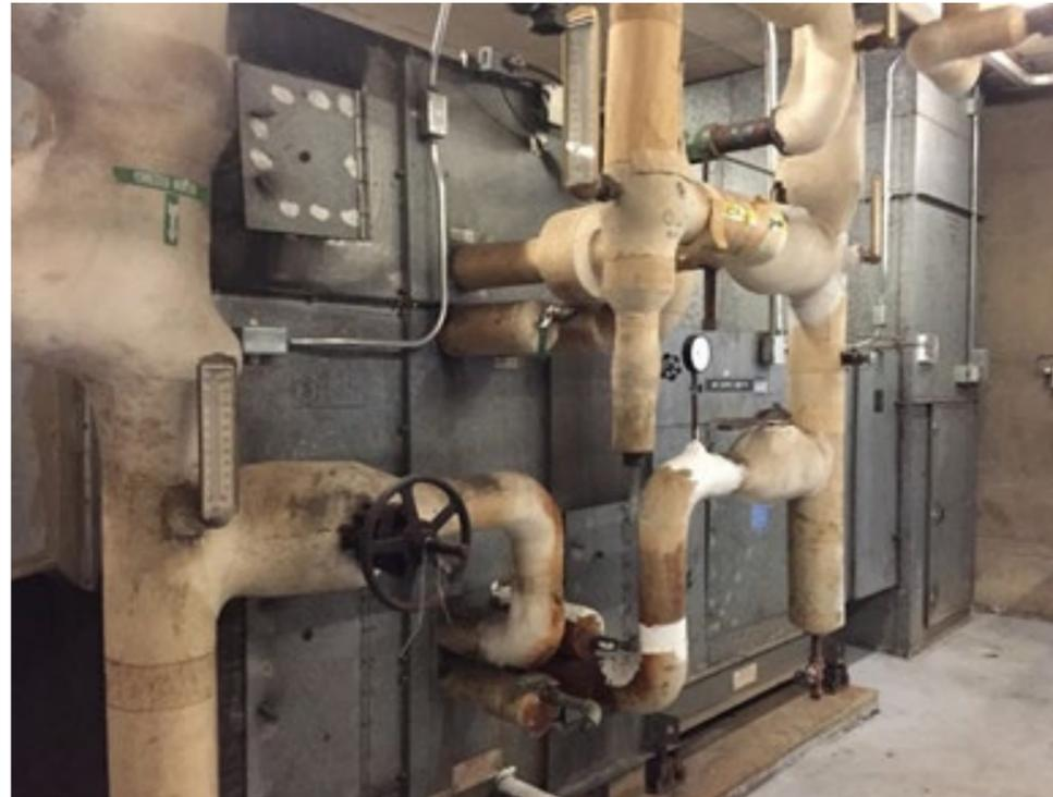
Figure 11 . Air handler (S-1) in Building A penthouse
