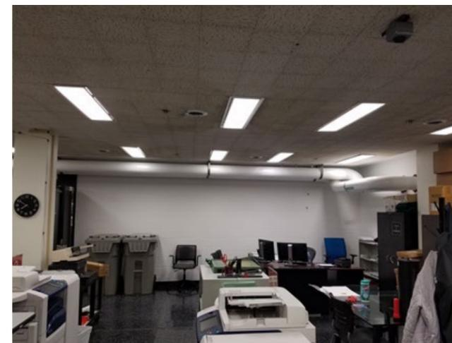
Figure 17 . Original integrated lighting and diffuser fixtures
