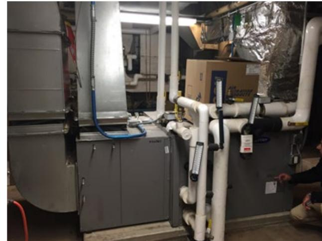
Figure 12 . Newly installed AHU-2 serving server room
