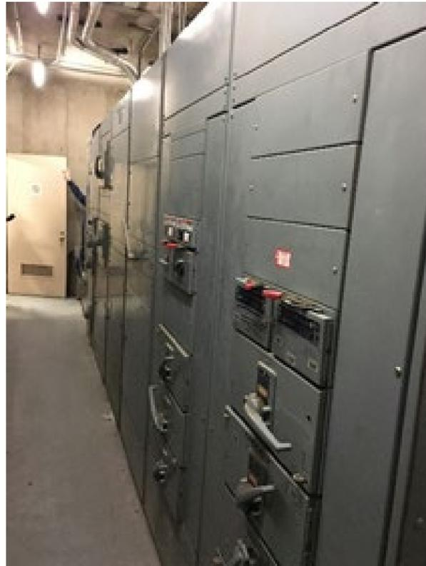
Figure 16 . Main switchgear
