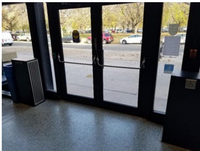
Figure 15 . Door heaters at ground floor main entrance
