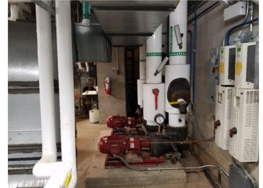
Figure 5 . Chilled water pumps installed in 2015
