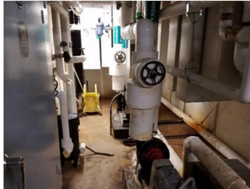
Figure 4 . Dual heating hot water pumps
