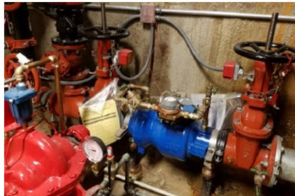
Figure 2 . RPZ installed in 2016
