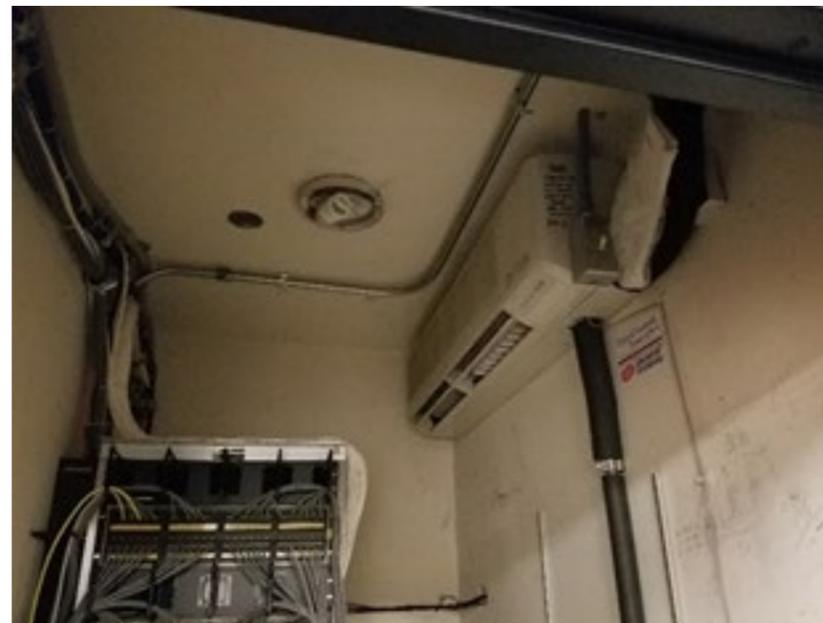
Figure 6 . Electrical room split system cooling unit
