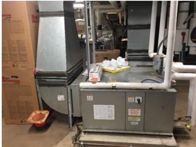
Figure 11 . Newly installed AHU-1 serving computer and conference rooms
