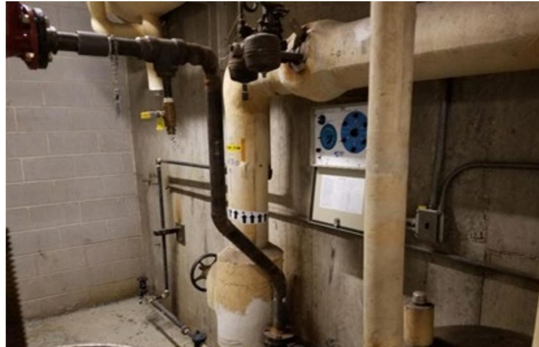
Figure 4 . Steam entry to basement mechanical room
