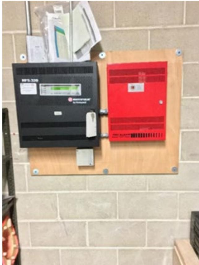
Figure 28 . Fire alarm control panel
