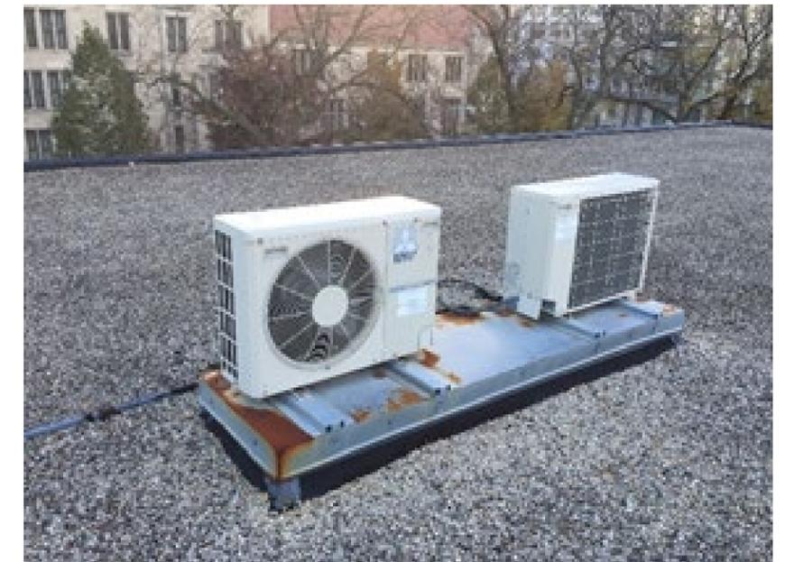
Figure 7 . Split system condensing unit on roof
