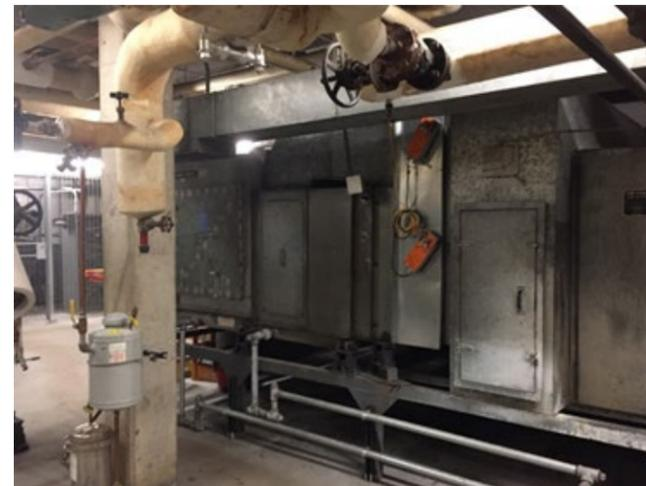
Figure 14 . Air handler (S-3) in basement mechanical room
