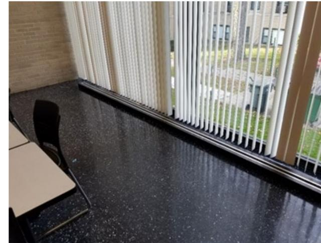
Figure 13 . Perimeter hydronic heating
