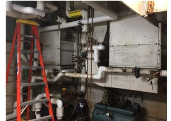
Figure 14 . Steam coils serving east and west door heaters
