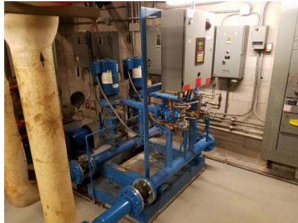
Figure 1 . Domestic water booster pump
