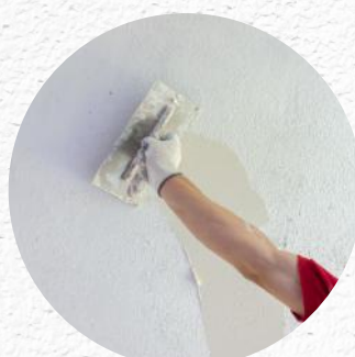
Internal plastering of walls & ceilings
