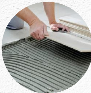
For Internal tiling application on floors
