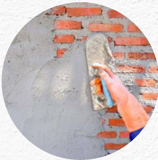
External plastering of walls
