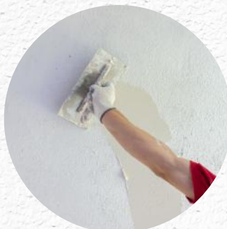
Internal plastering of walls & ceilings
