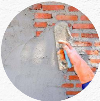
External plastering of walls
