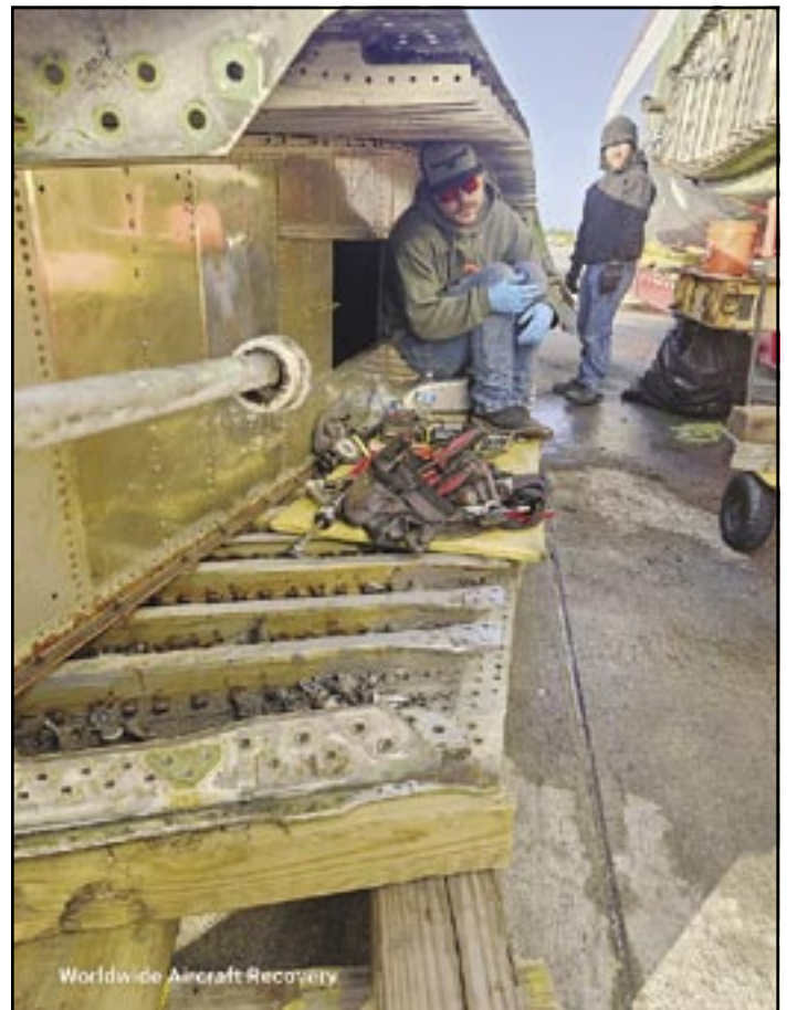
ABOVE: A confined space to work in.
