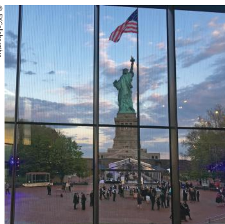
The New Statue of Liberty Museum uses low-reflective insulated glass with an original frit pattern to deter bird collisions.
