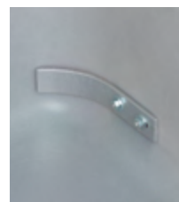
Platform fastening (reinforcement)
