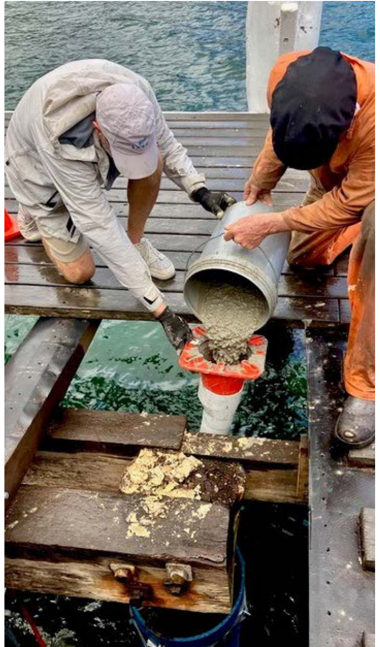
Pouring the cement. Photo Chris Manion
