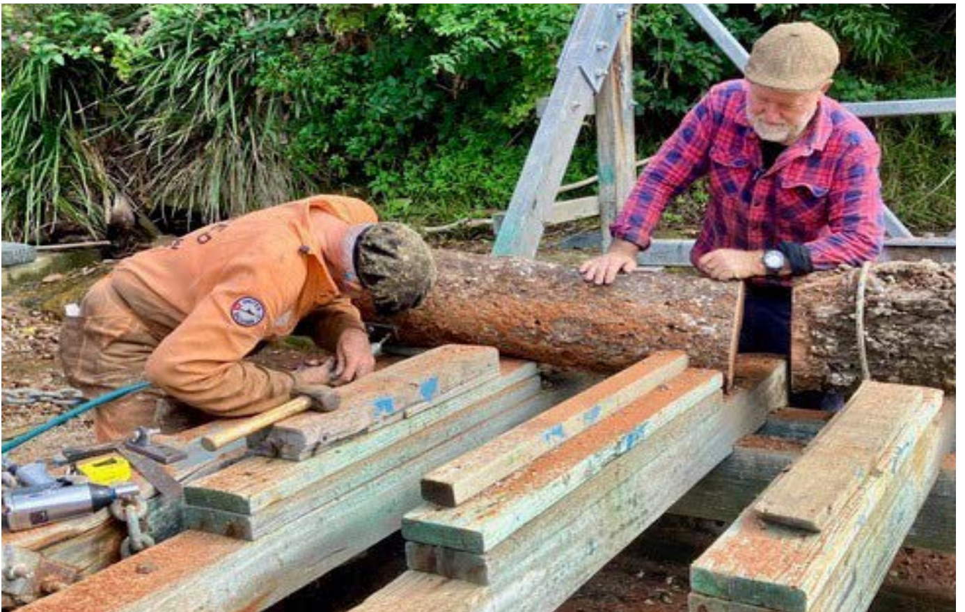
22 Bruce and Trevor measuring a new pile. Photo David Salter
