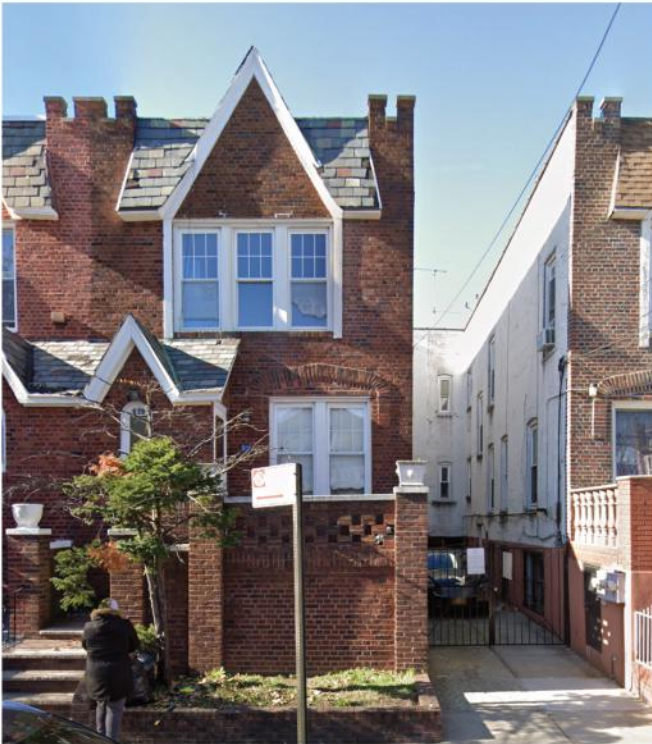
FRONT ENTRY PHOTOGRAPH OF 704 E 51ST STREET
