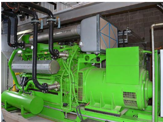
Biogas systems produce electricity by burning biogas in a co-generation system. (Image: https://www.ontario.ca/page/anaerobic-digestion-basics )
