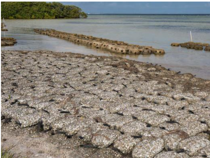
Living shoreline restoration project, Tampa Bay, FL. Oyster reef balls, marsh grass and bagged fossilized shell. (Image: Shutterstock 2287295785)
