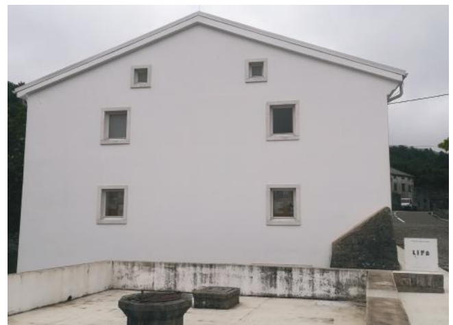
Above, the village of Lipa and an exterior view of the museum | EUROM
