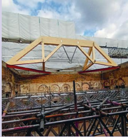
Above Steel-braced glulam trusses span a square opening to create the imposing new faux rooflight.
