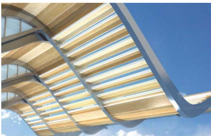
The louvres on the canopy allow light and air to filter in, creating bright and airy spaces.
