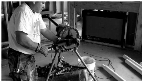
(Figure 1). Cutting End of Pipe
