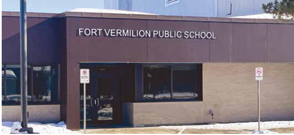
The solution was to expand and modernize the existing Fort Vermilion Public School, located on higher ground outside the flood zone, into a shared space for both schools.
