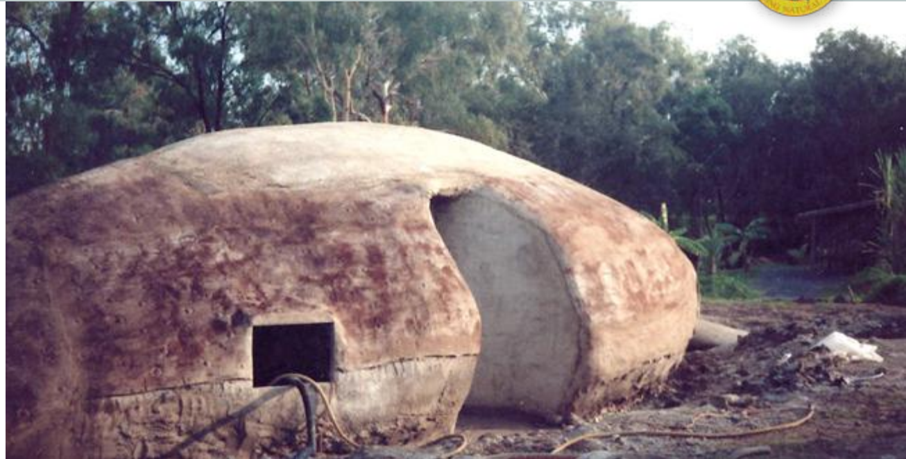
Entry with sprayed concrete before smoothing
