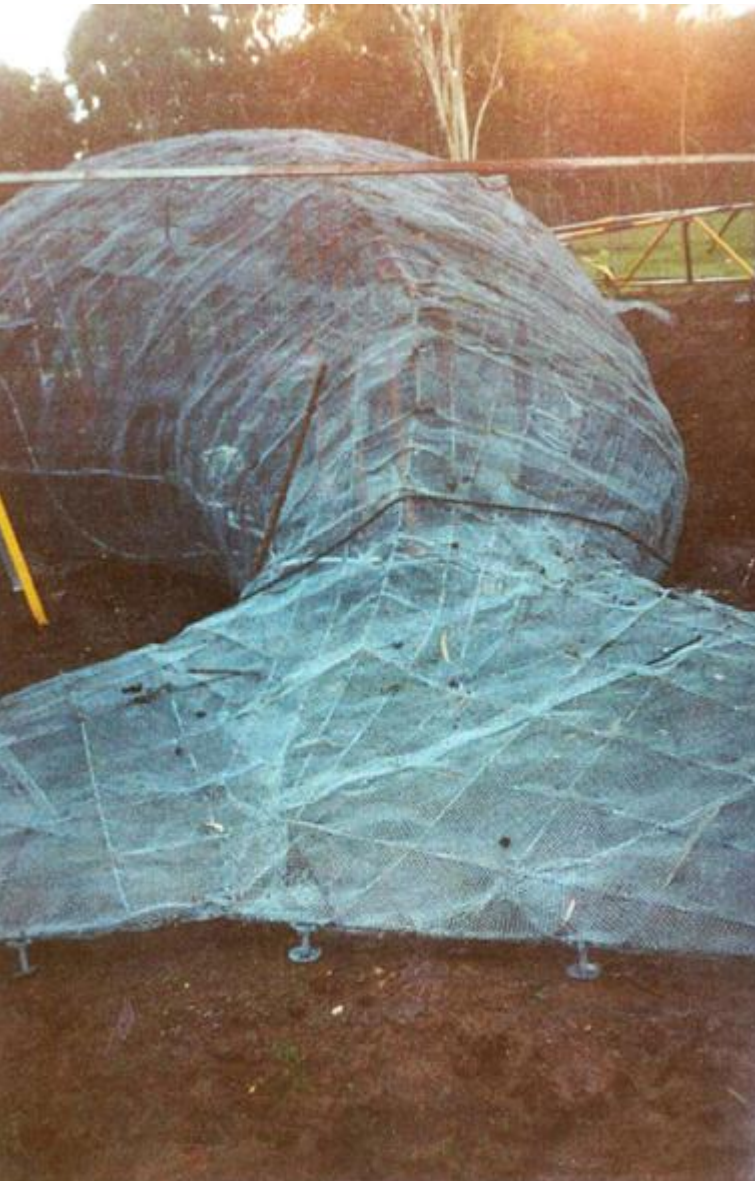
Covering with wire mesh, raising off the ground slightly
