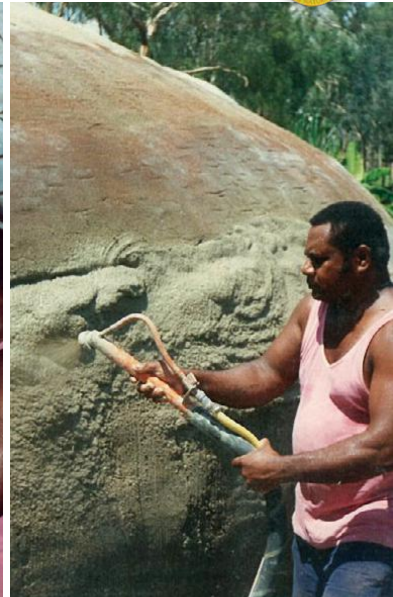
Spraying external mesh frame with concrete
