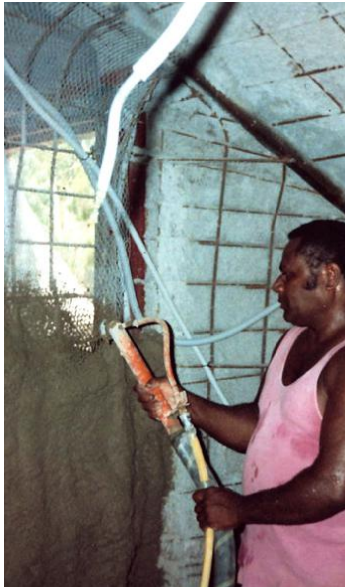
Spraying internal mesh frame with concrete. Layering step by step
