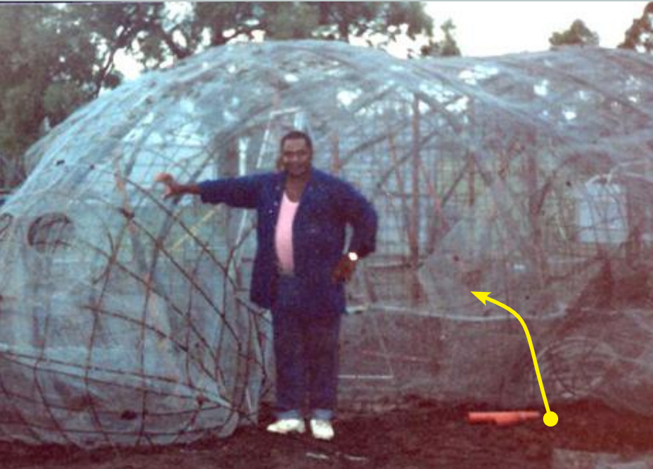
Steel armature with wire mesh
