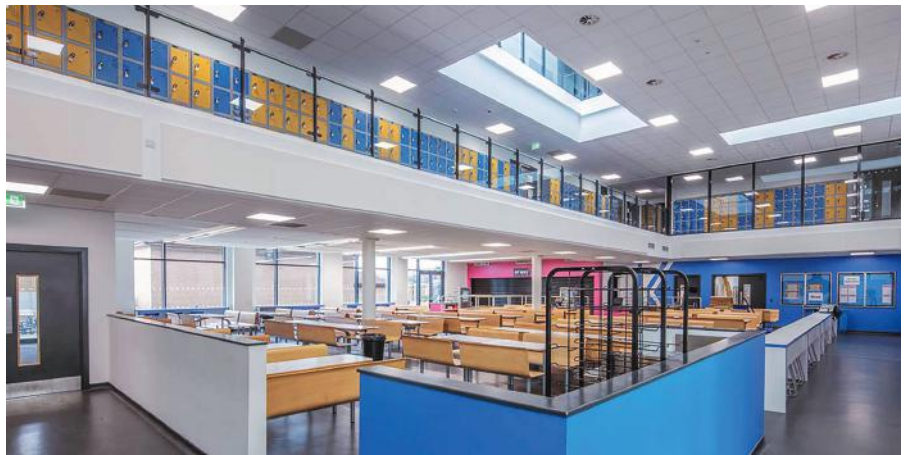
Heat emitters were upgraded to be future-ready for installation of heat pumps
