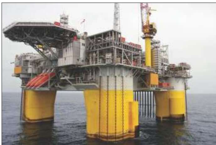
Polyester coatings, particularly those with glass flakes, excel in harsh environments such as splash zones of offshore structures.
