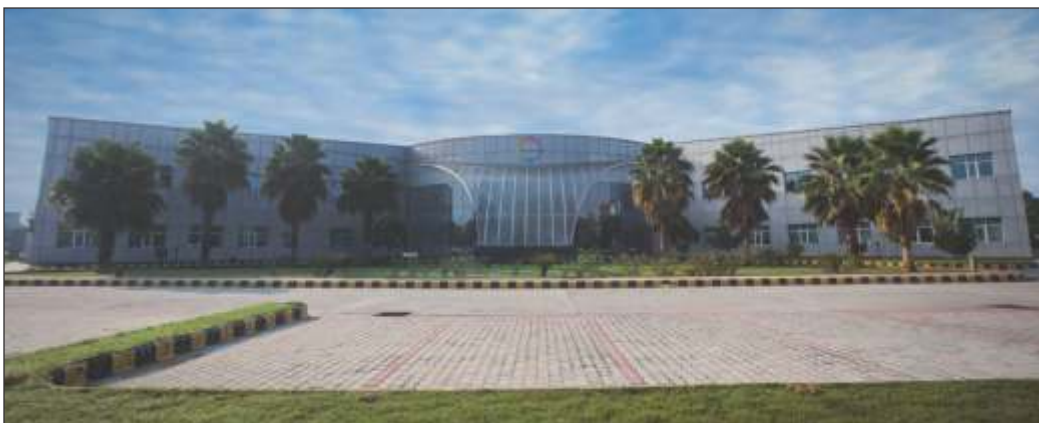
The Covestro facility in Greater Noida, one amongst the many in India.
