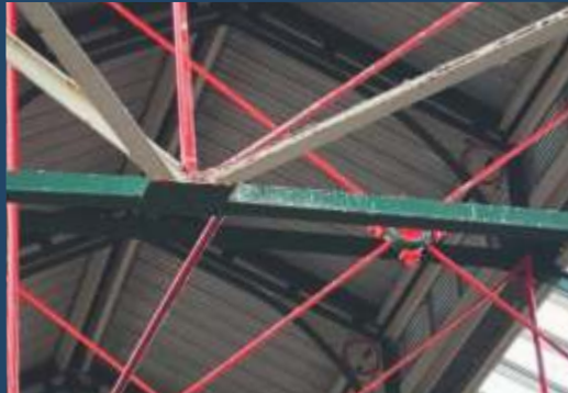
Mild steel substrate with aluminium rich epoxy primer containing zinc phosphate + topcoat
