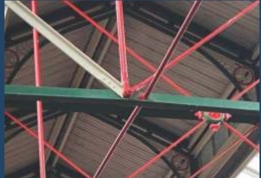
Mild steel substrate with aluminium rich epoxy primer containing zinc phosphate & 5% Intelli-ion® + topcoat
