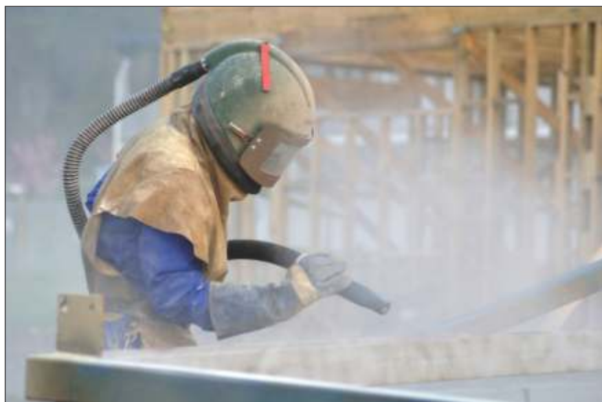
The best surface preparation involves achieving a blast-cleaned surface with a Sa2½ finish, accompanied by a suitable anchor profile.
