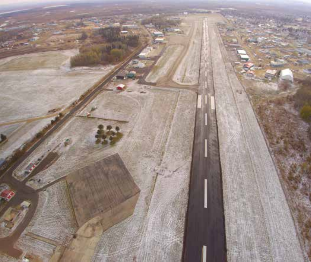
OLS exists to protect the airspace around airports for arriving and departing aircraft, as well as for circuit flying and missed approaches.
