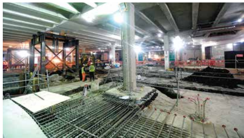
New reinforcement to piles and table frame supporting ground floor slab during column replacement.
