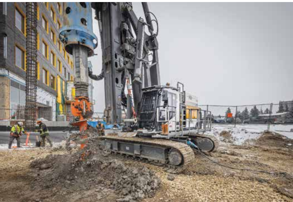
The LB 30 unplugged installed 22 piles using the Kelly method.
