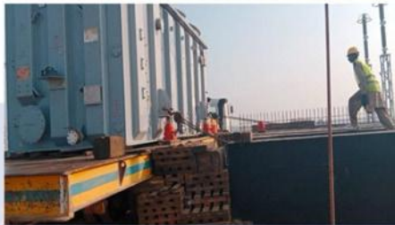
Manual Unloading & Placement of Transformer on foundation via jacking & skidding process
