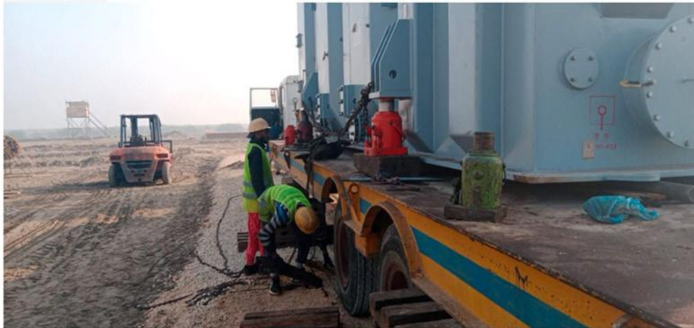
Manual Unloading & Placement of Transformer on foundation via jacking & skidding process
