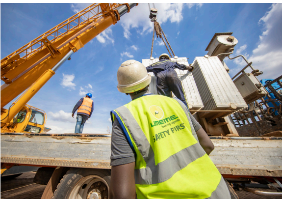
Loading transformer ahead of a field installation
