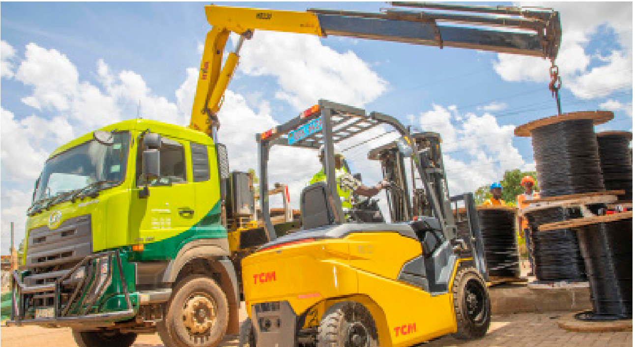
Engineering teams assembling cables ahead of a field excursion.
