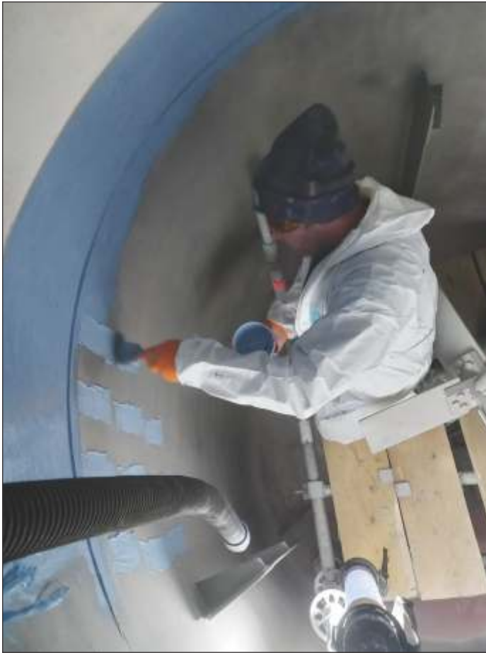
Figure 3: Application of high-performance coating, Belzona 1391T.
