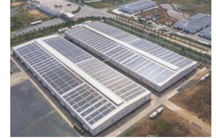
Long An Int. Port Warehouses
