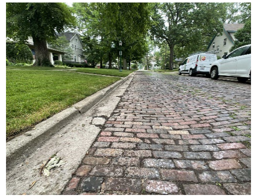
Edge After Repair
