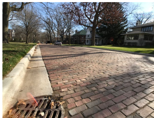
Brick Paver Reconstruction
