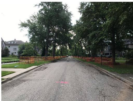
Existing Asphalt Overlay
