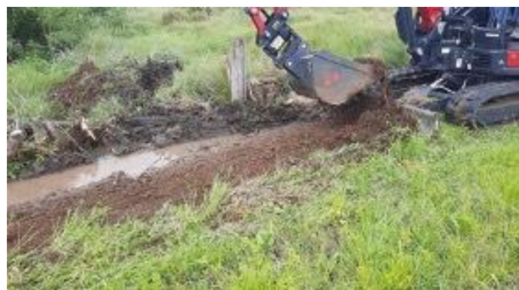
At least the digging in soft soil was relatively easy, although only suited to lighter weight machinery with the risk of getting bogged.
