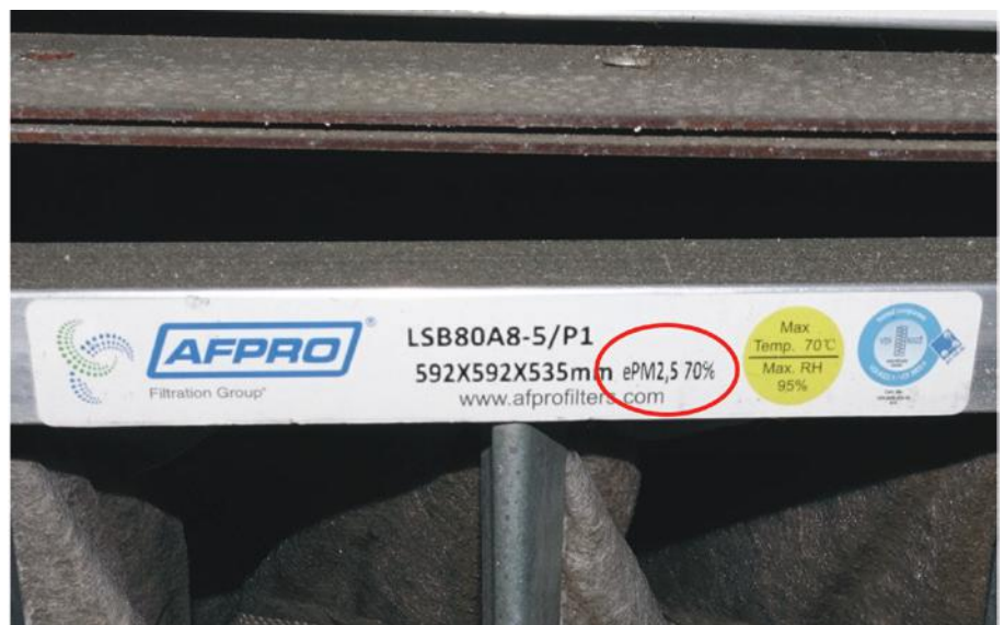
Figure 6 – Example of a filter label applying the ISO16890 classification
