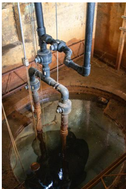
Kensa System drawing water from the Taff's Well thermal spring
