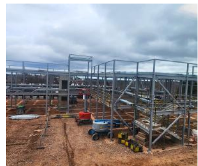
Phase 2 Steel Frame
