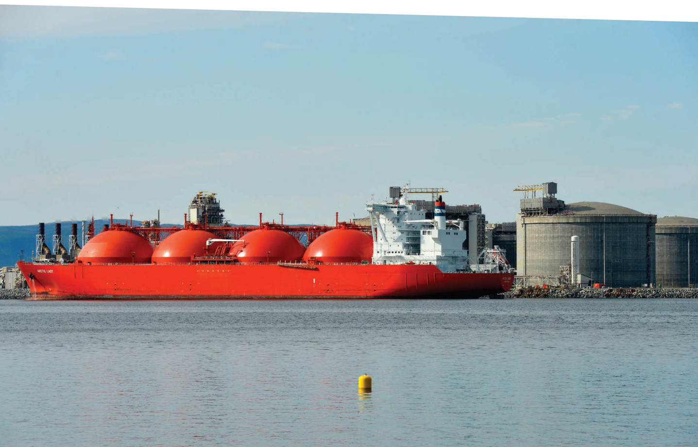
Hammerfest LNG plant at Melkøya. Foto Harald Pettersen/Equinor
