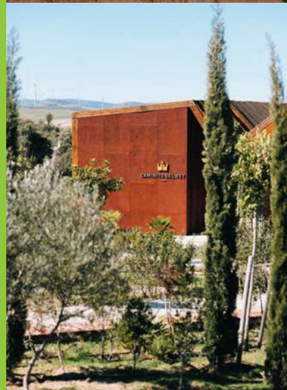
Far top to bottom The new Caminito path is located above the original one; the starting point of El Caminito Del Rey; all walkers have to wear helmets on the trail
