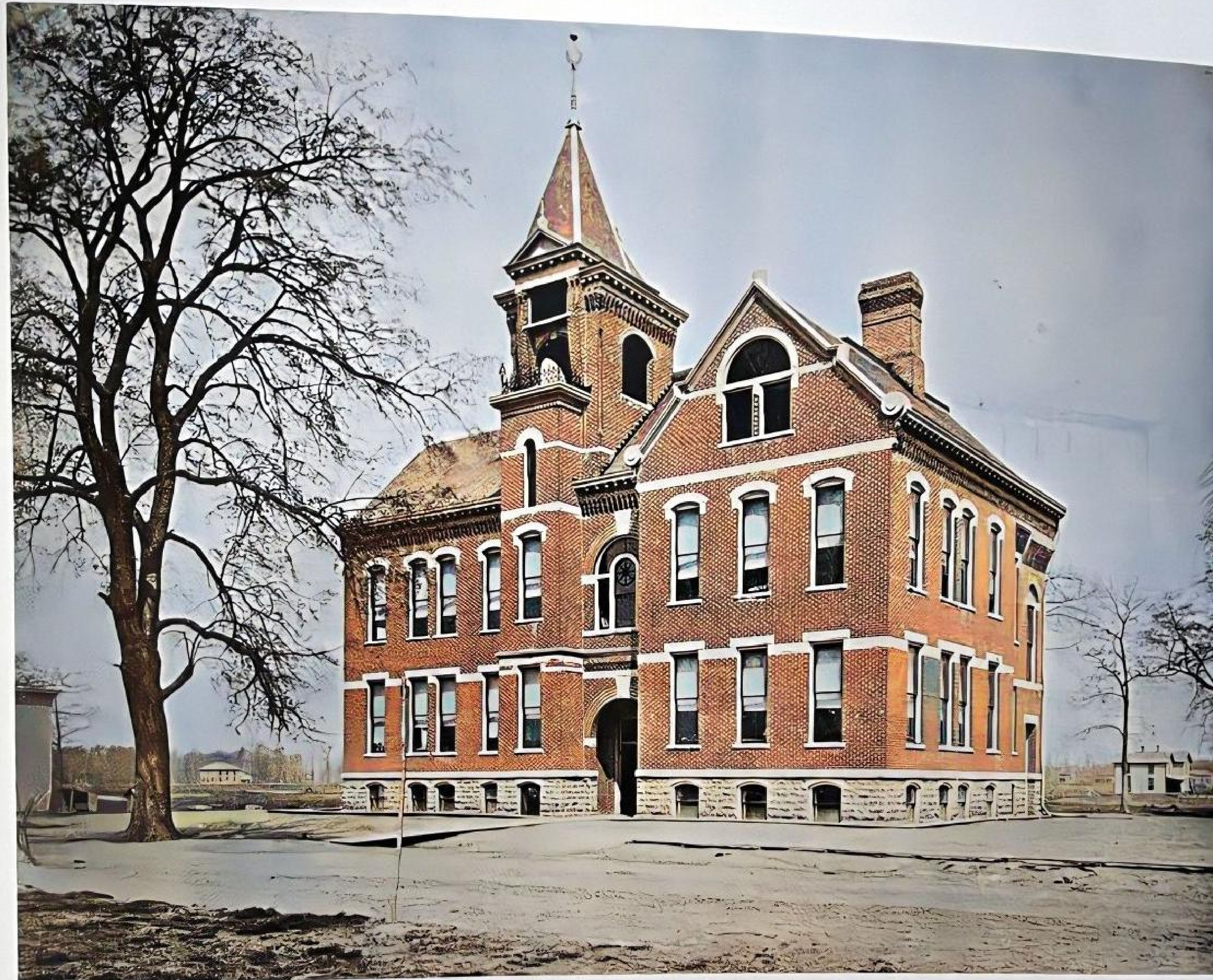
HOWARD SCHOOL—ONE OF FIVE NEW SCHOOL BUILDINGS.
