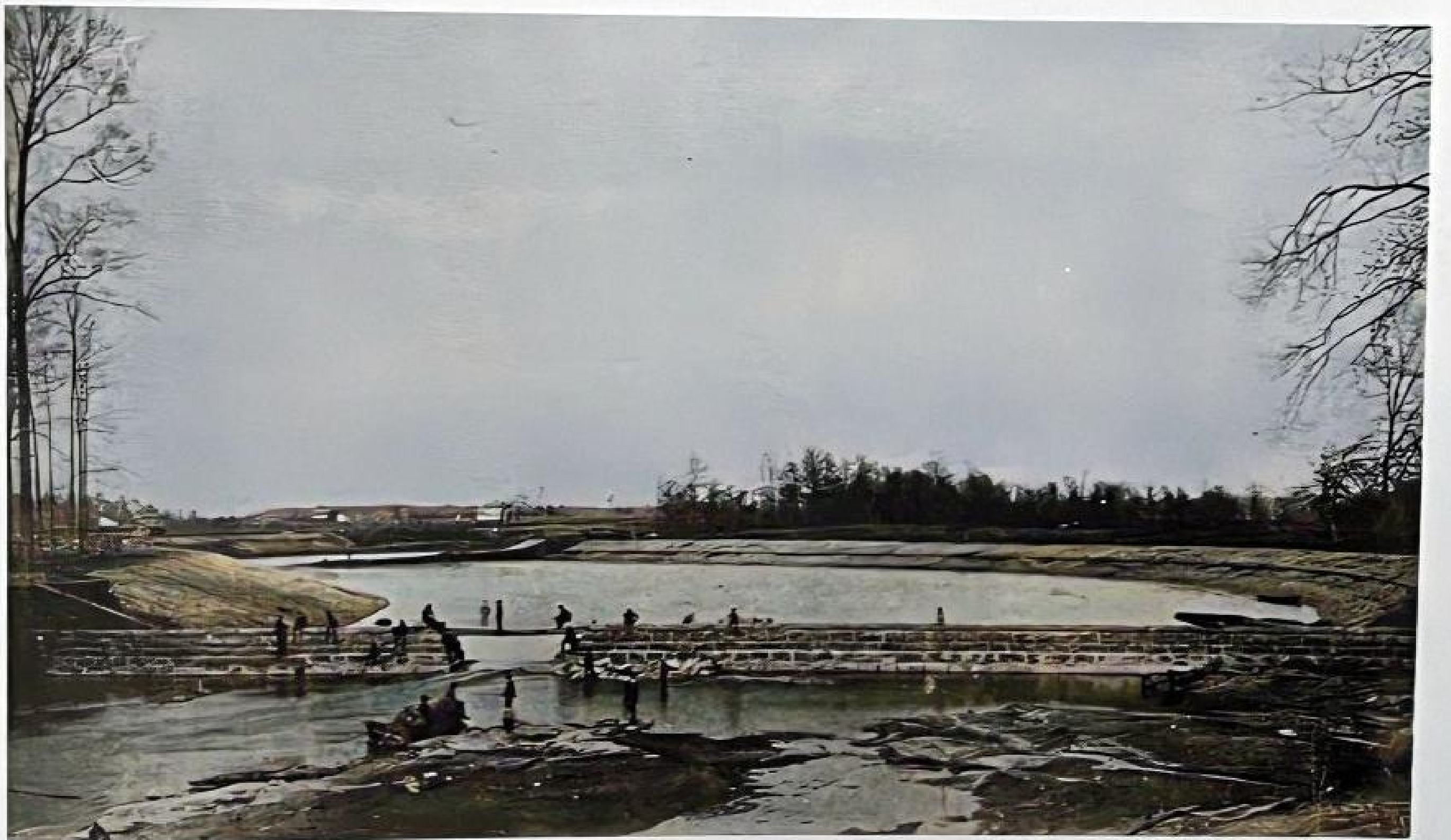
VIEW OF MASONRY DAM, FINDLAY WATER WORKS.
