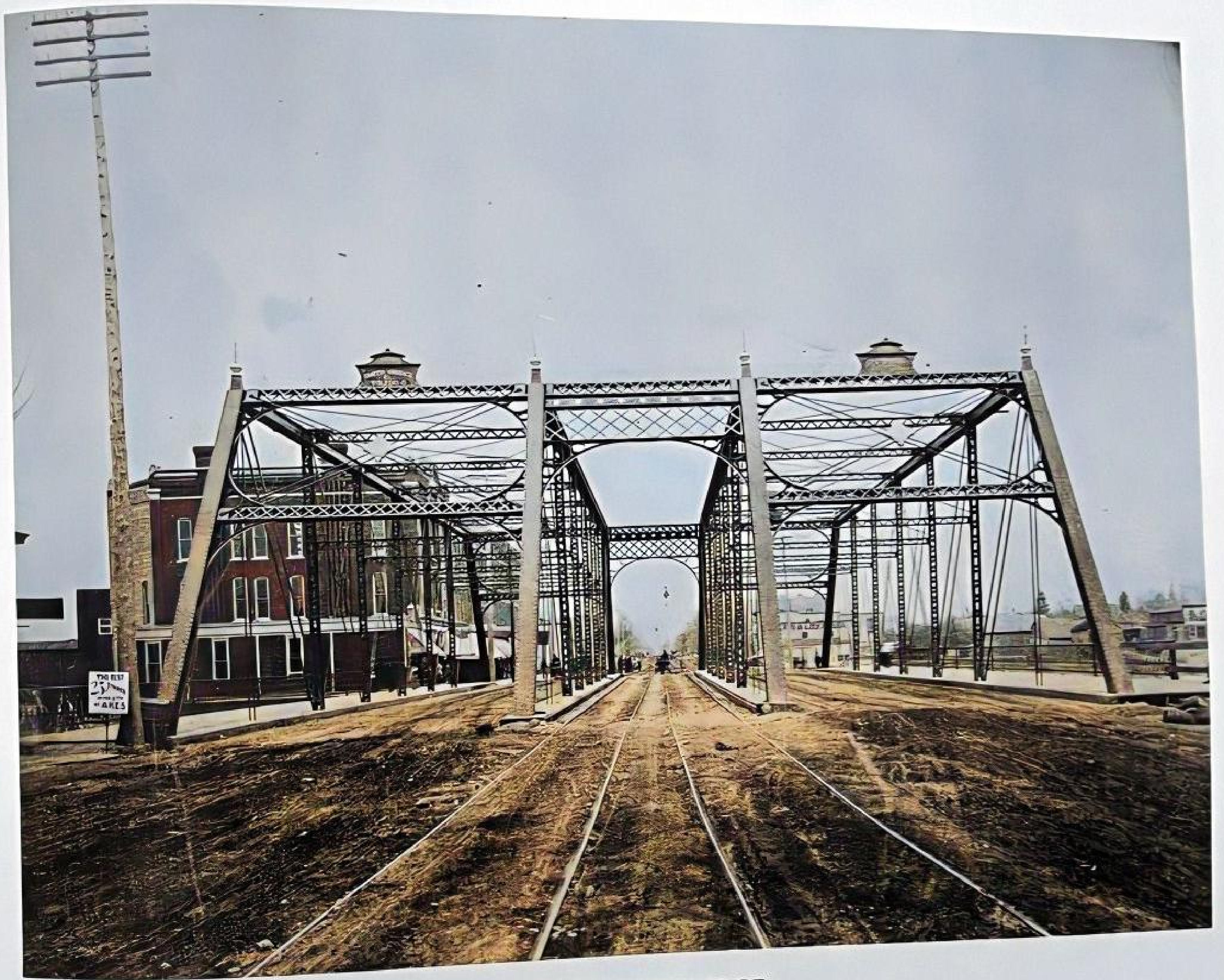
MAIN STREET BRIDGE.
