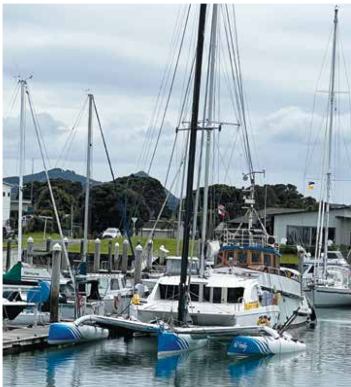
Marsden Cove Marina, with port float damage evident
